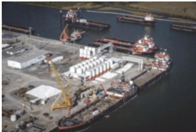
HOS Port Facility in Port Fourchon Louisiana
